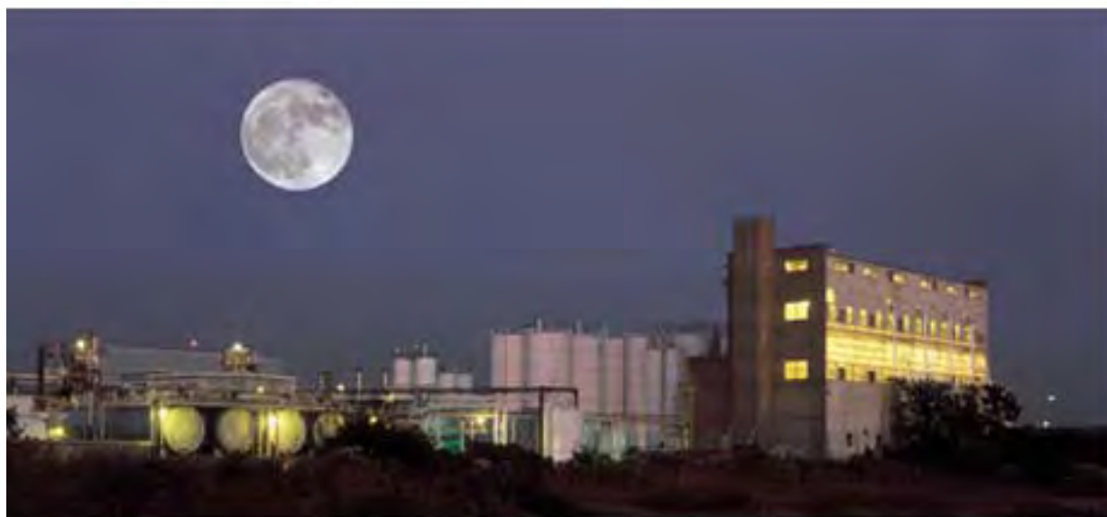
Chesapeake, VA Styrenics Facility
