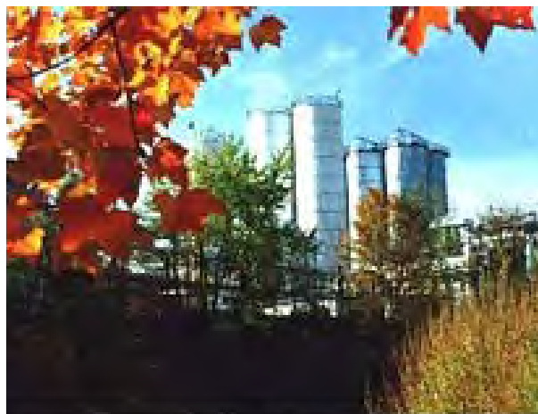
Indian Orchard, MA Styrenics Facility
